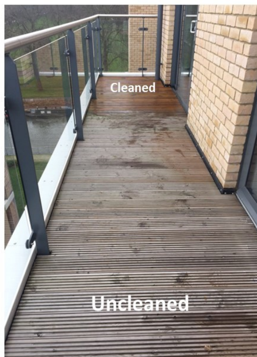
Wood decking being cleaned prior to protection
