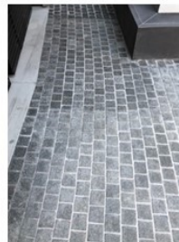
Basalt Pavers after cleaning with ConClear to remove cement residue
