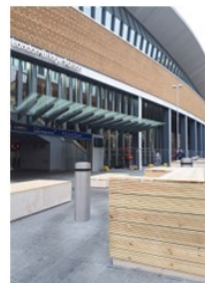
Basalt Pavers after cleaning with ConClear to remove cement residue
